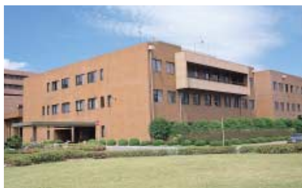
管理棟 Administration Building
