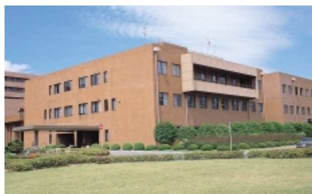
管理棟 Administration Building
