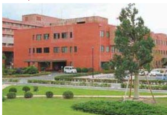
管理棟 | Administration Building
