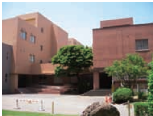
建物全景生物資源開発部門(左)と放射性同位元素利用部門(右) | Buildings of the Divisions of Biological Resources and Development (Left) and Radioactive Compounds Utility (Right).
