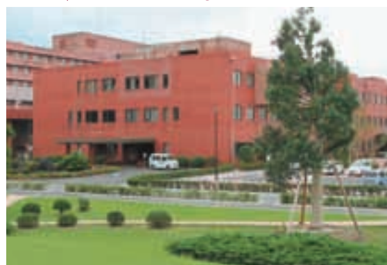
管理棟 | Administration Building
