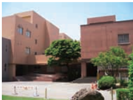
生物資源開発部門(左)と放射性同位元素利用部門(右) | Buildings of the Divisions of Biological Resources and Development (Left) and Radioactive Compounds Utility (Right).
