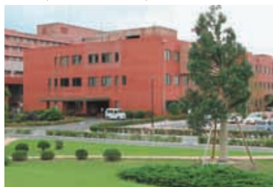
管理棟 | Administration Building
