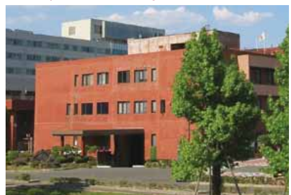
管理棟 | Administration Building
