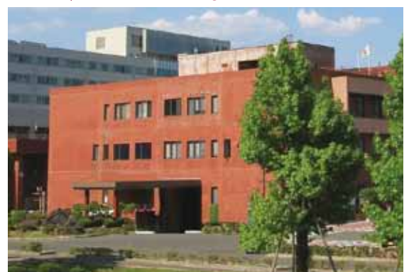
管理棟 | Administration Building
